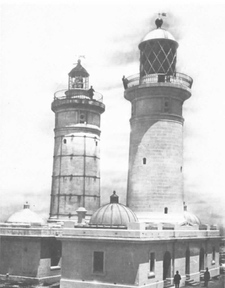
In 1883 the present Macquarie Light replaced the old convict-built tower which, by that time, was bound together by iron hoops.
