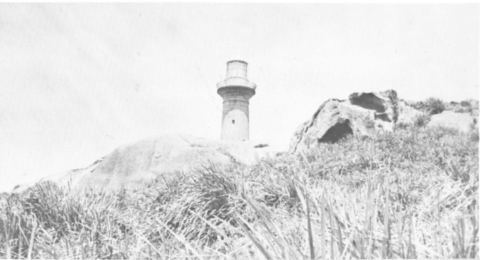
The 69-ft. tower of Montagu Island light stands a total of 262 feet above high water and has a range of 20 miles.
