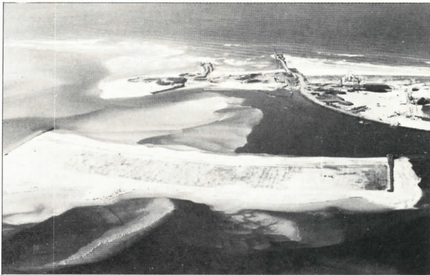
The new entrance under construction with Wave Break Island in foreground.
